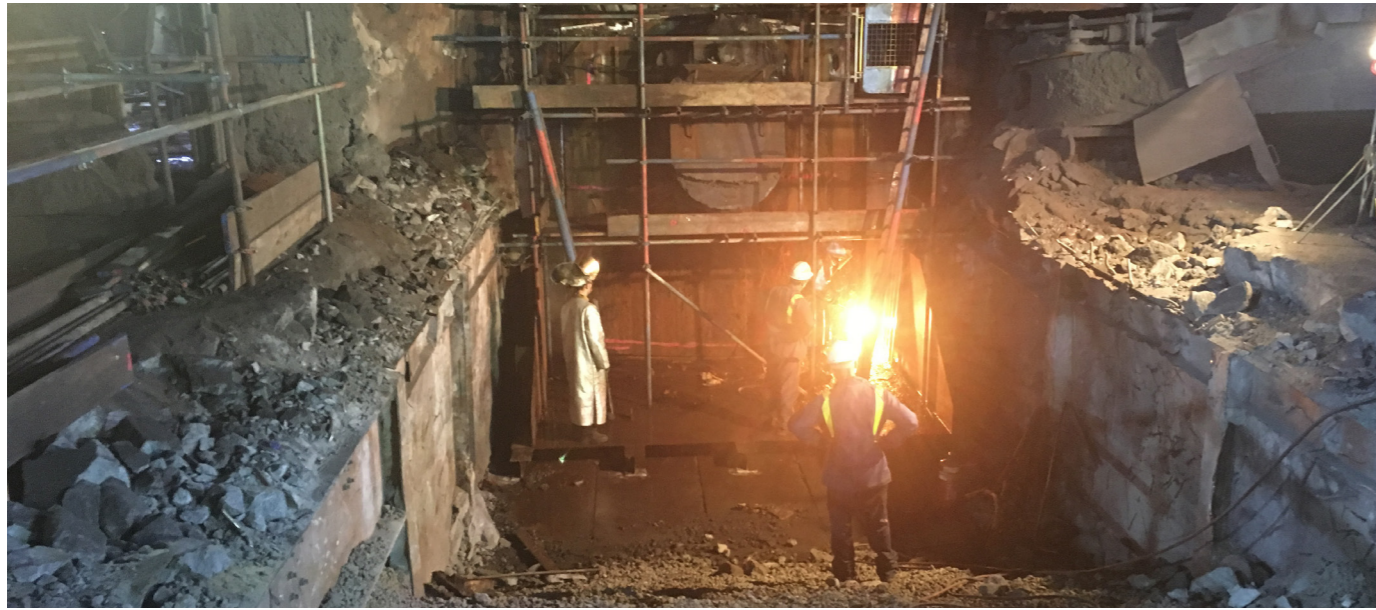
Tata Port Talbot No.5 Blast Furnace. Preparing to breach the furnace
