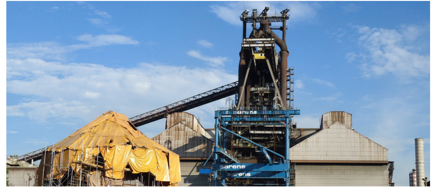
ArcelorMittal Tubarão No.1 Blast Furnace. Shell pre-assembly and gantry system
